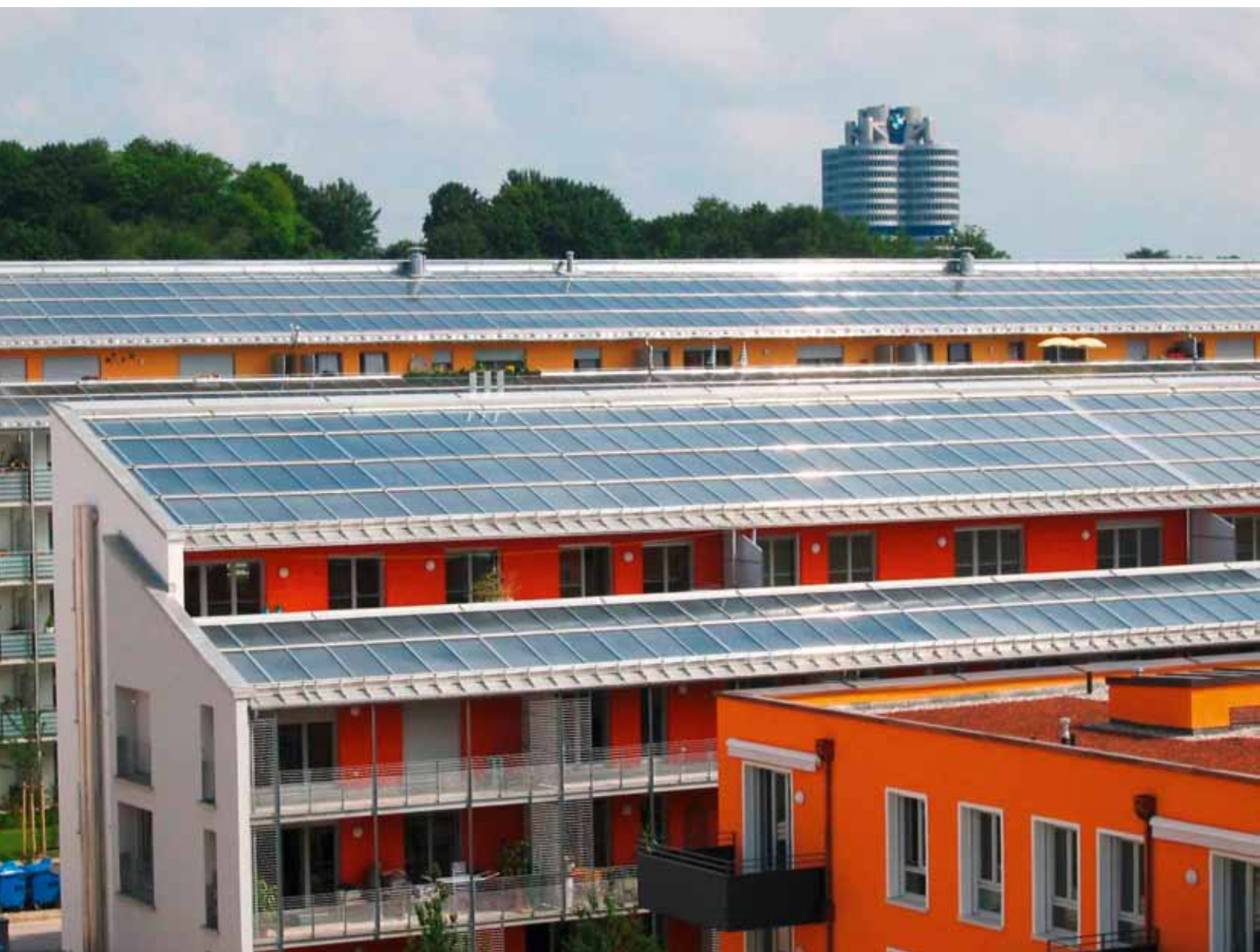
Large-scale solar heating at Ackermannbogen / Munich
